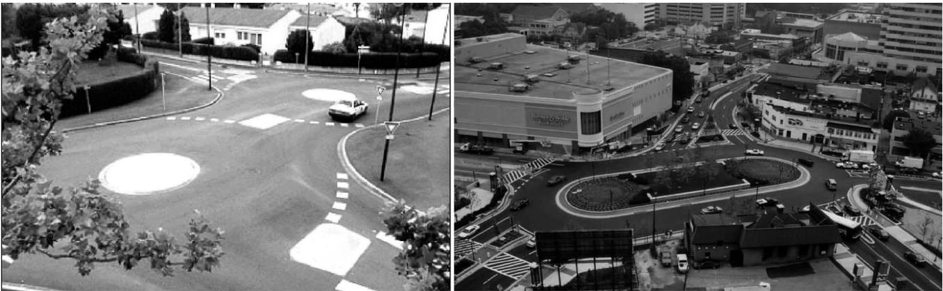
Figura 7 - (a) Rotunda dupla / (b) rotunda alongada (<http://www.ksu.edu/roundabouts/>; / [www.trans.ci.portland.or.us](http://www.trans.ci.portland.or.us))
